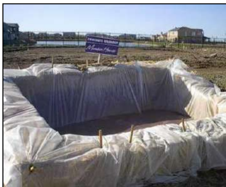
Plate 3-1 Typical concrete wash out areas
