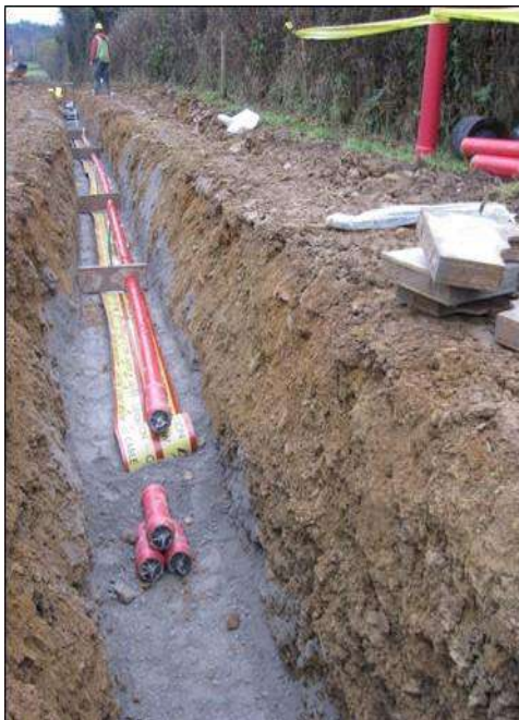
Plate 3-4: Typical Cable Trench View
