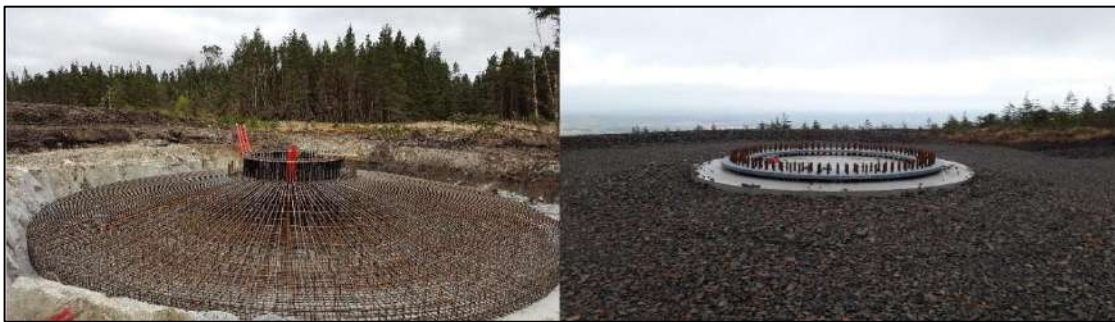
Plate 3-2: Turbine 'Anchor Cage' and finished turbine base
