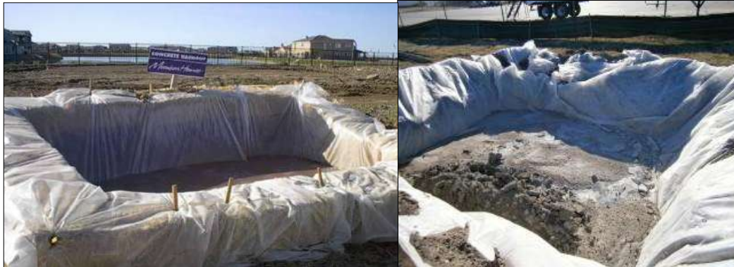
Plate 3-3: Concrete washout area
