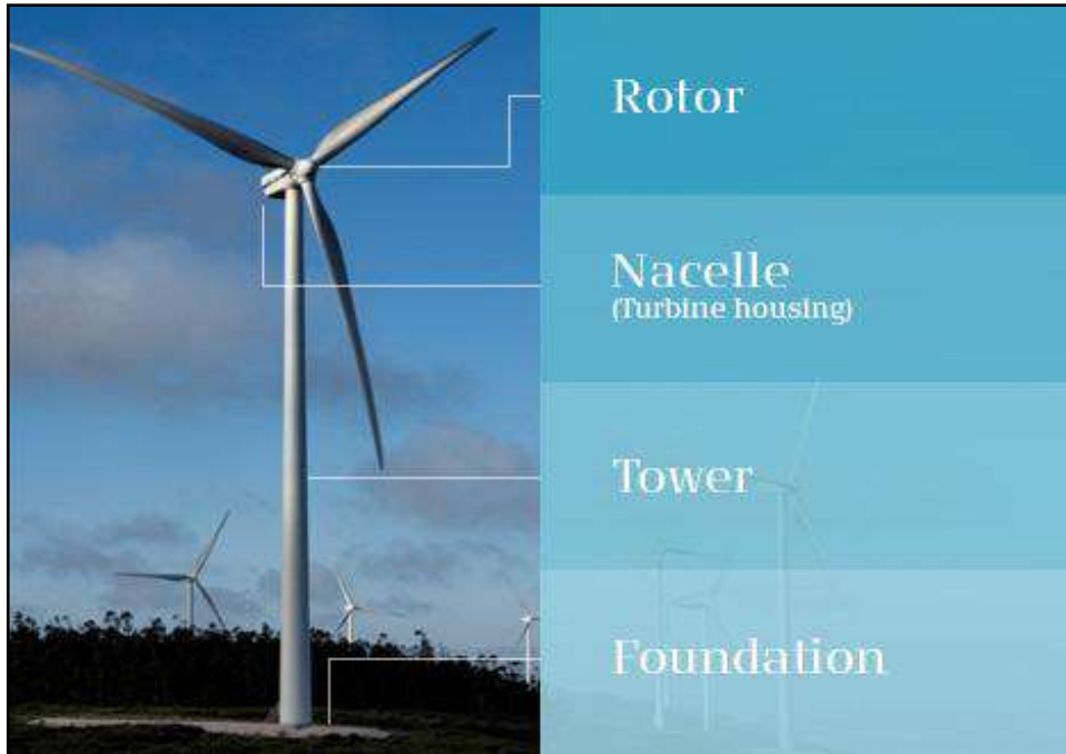
Plate 3-1 Wind turbine components
