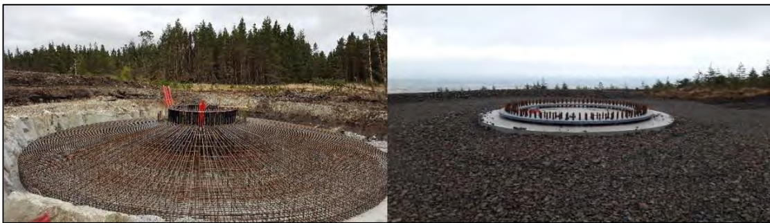
Plate 3-2: Turbine 'Anchor Cage' and finished turbine base
