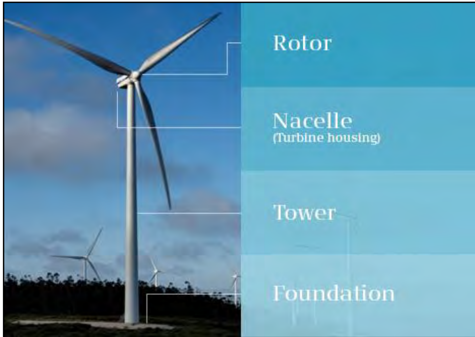
Plate 3-1 Wind turbine components
