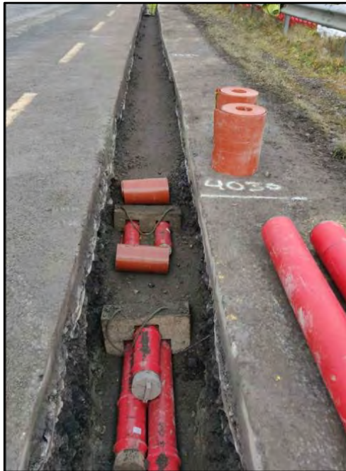
Plate 2-1 110Kv Cable Trench View
