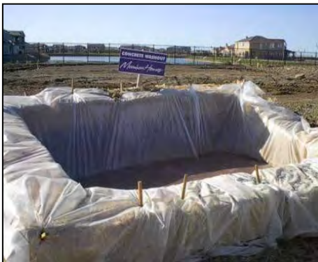
Plate 3-1 Typical concrete wash out areas
