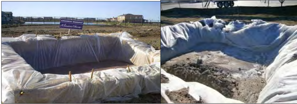
Plate 4-3 Concrete washout area
