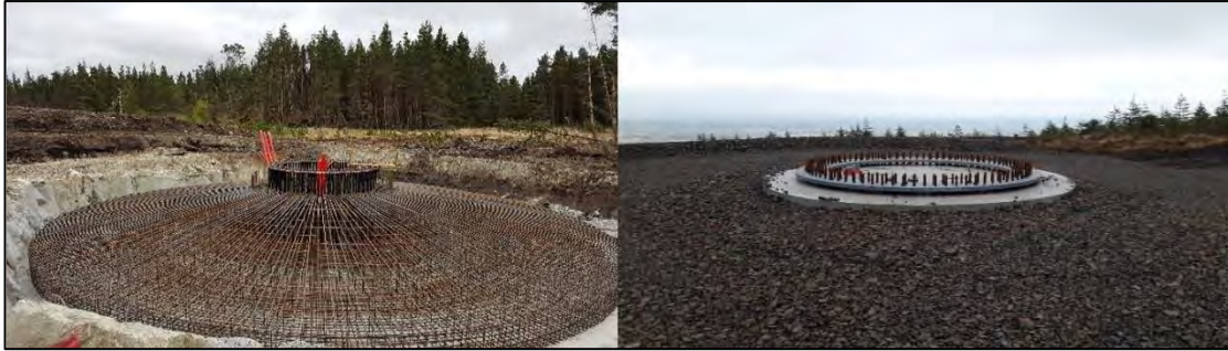
Plate 4-2 Turbine 'Anchor Cage' and finished turbine base
