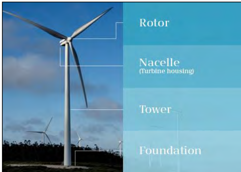
Plate 4-1 Wind turbine components
