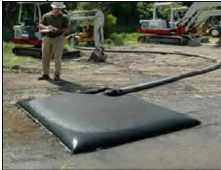
Plate 4-5 Silt Bag with water being pumped through
