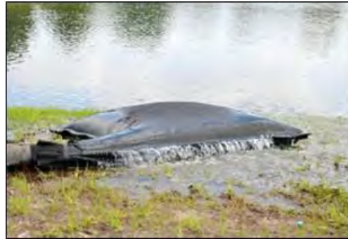
Plate 4-6 Silt bag under inspection
