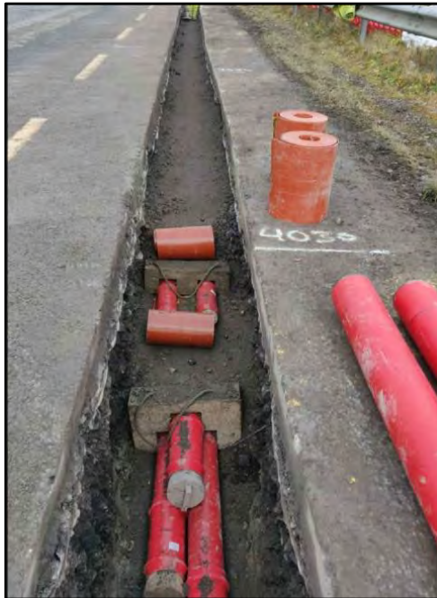
Plate 2-1 110Kv Cable Trench View
